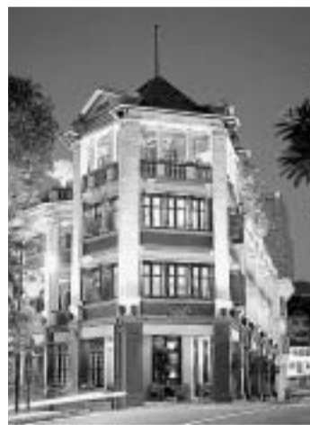
Glamorous: the hotel facade.
